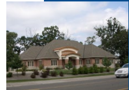
These examples of suburban commercial development along Drake Road and Stadium Drive have a wide landscaped greenway that screens the parking from the arterial road.
