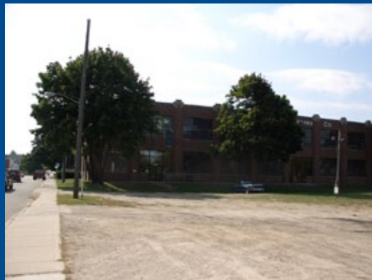
This former factory has been adaptively reused for a number of different uses on Fulford
