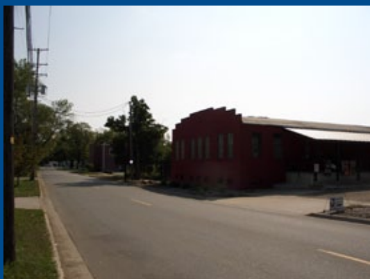
The Metals Studio just north of downtown is an excellent example of creative uses for former industrial buildings in Employment and Mixed-Use areas
